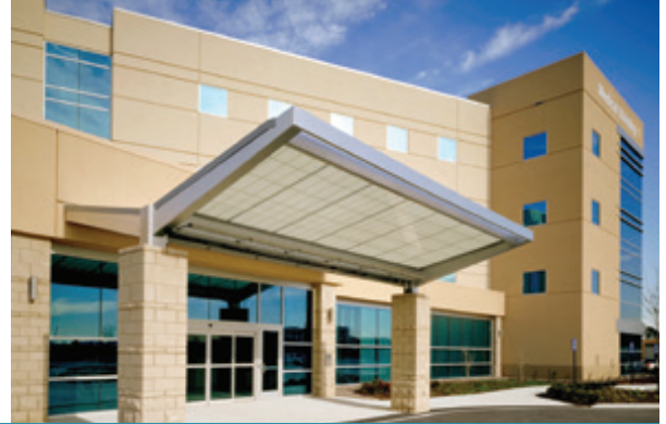
Denton Exterior Entrance
